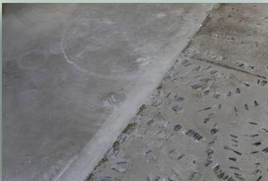
Here you can see a relatively good underfloor (on the left) and one that needs some treatment (on the right).
