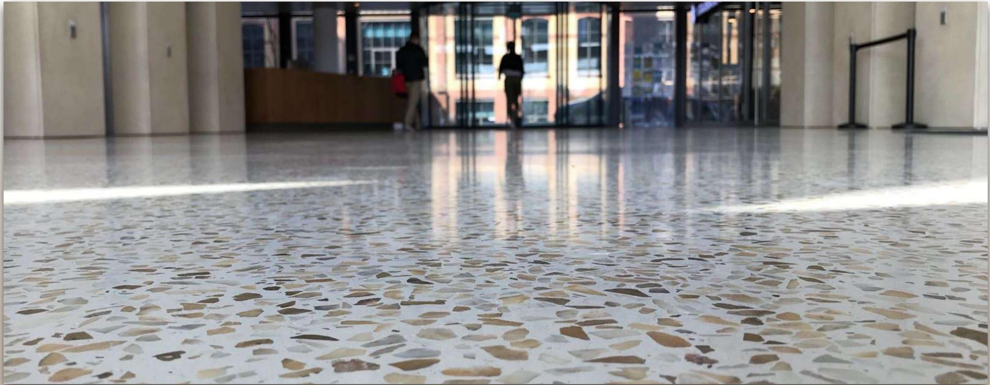
A two components mineral based screed, EPOXY FREE, that can be used to create uniform floors with micro or big aggregates exposure, ground and polished to the desired effect and result, entirely SEAMLESS and no joints!
